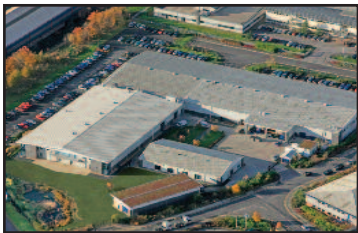
AESSEAL plc Group Headquarters, Rotherham, UK.
